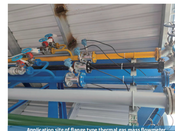
Application site of flange type thermal gas mass flowmeter
