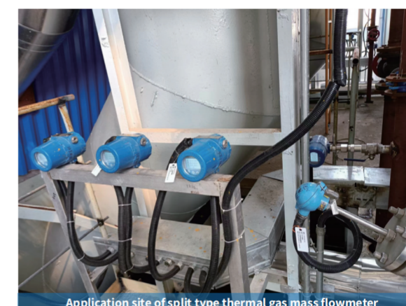
Application site of split type thermal gas mass flowmeter
