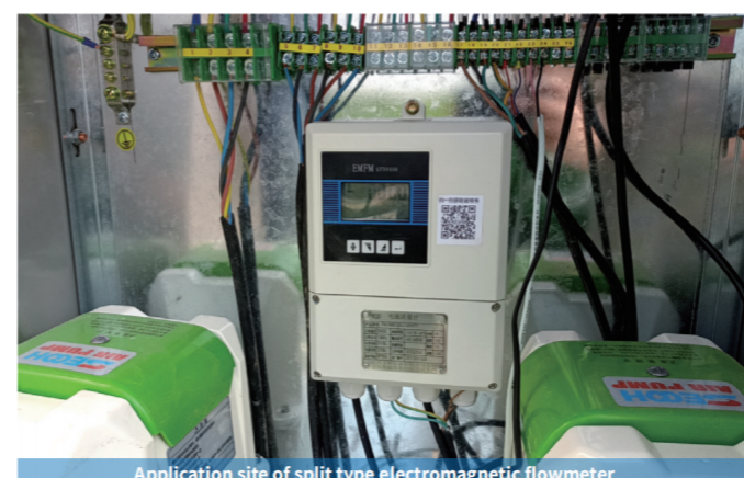
Application site of split type electromagnetic flowmeter
