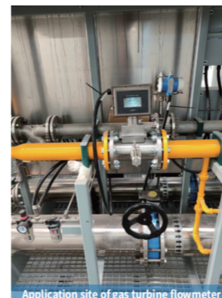
Application site of gas turbine flowmeter
